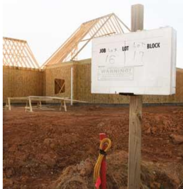
Outside plant cables, either aerial or underground, get closer to the home.
